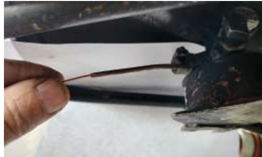
Introduce a probe wire through the copper water tube from the outside.
