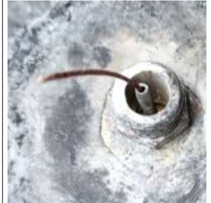
View from the inside the exit of the probe wire.
